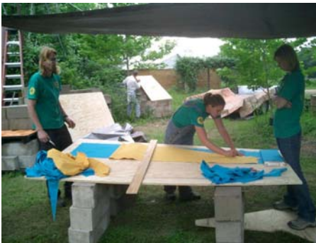
cutting roof fabric
