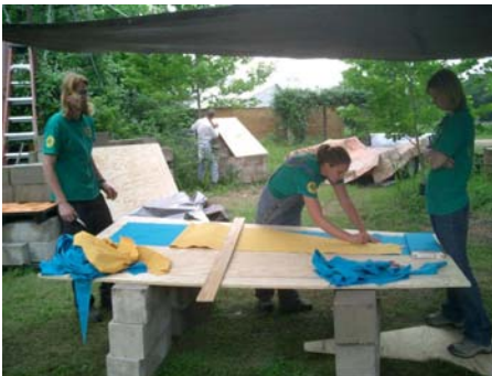
cutting roof fabric
